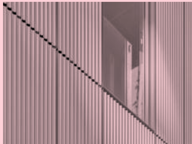
[09] FAÇADE CLOSE-UP VIEW OF 39 KING'S ROAD © XU LIANG LEON 2023
