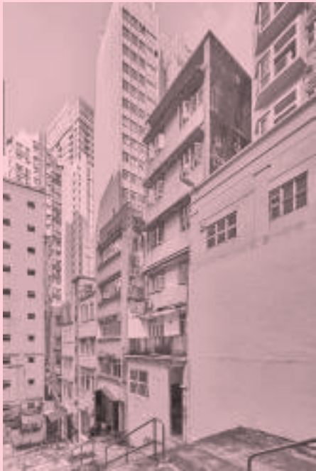
[10] FAÇADE VIEW OF 10 SIK ON STREET BUILDING BEFORE RENOVATION, HONG KONG © XU LIANG LEON 2019
